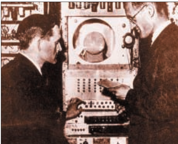
Freddie Williams and Tom Kilburn and 'The Baby', which had a cathode ray tube memory
